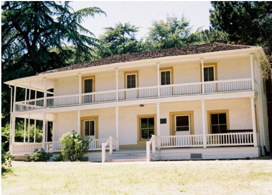
The Martinez Adobe is one of the small number of structures in California dating back to Statehood and beyond. Constructed circa 1849, the building has been seismically retrofitted, and should now last the ages. It is currently displaying the first full scale exhibit on the historic de Anza Trail.
