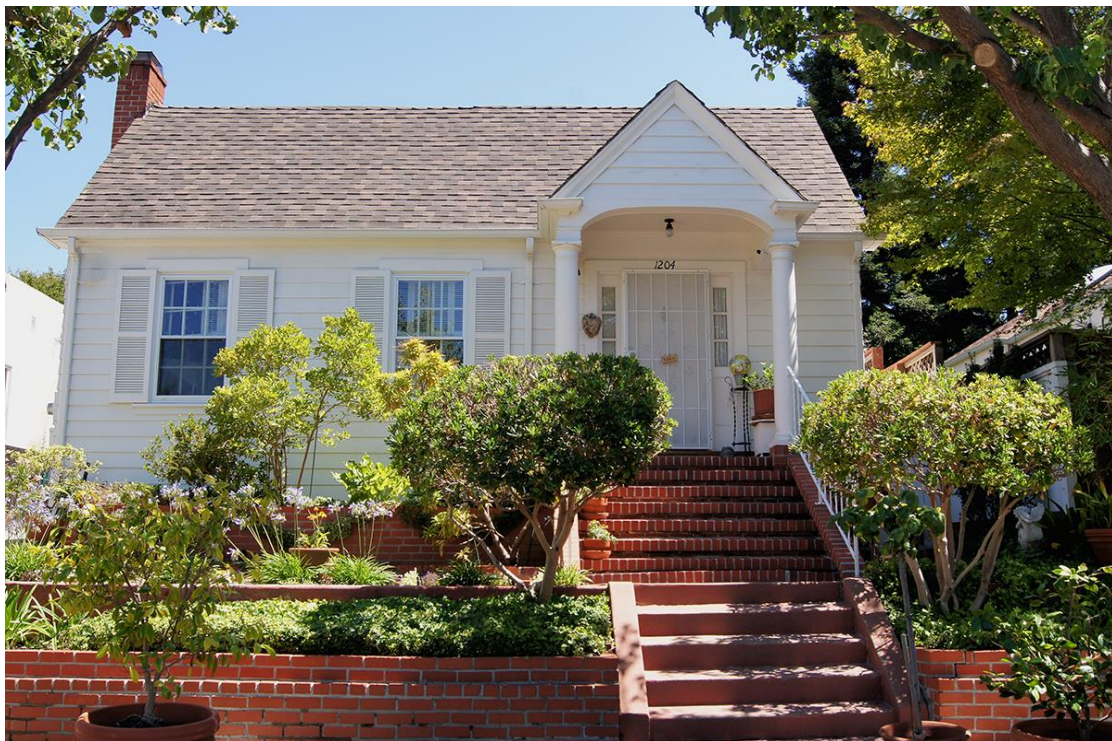
This Colonial Revival home is entered via a classic portico supported by two columns.
